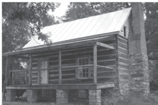
2007 ~ Restored Holland Page Place
